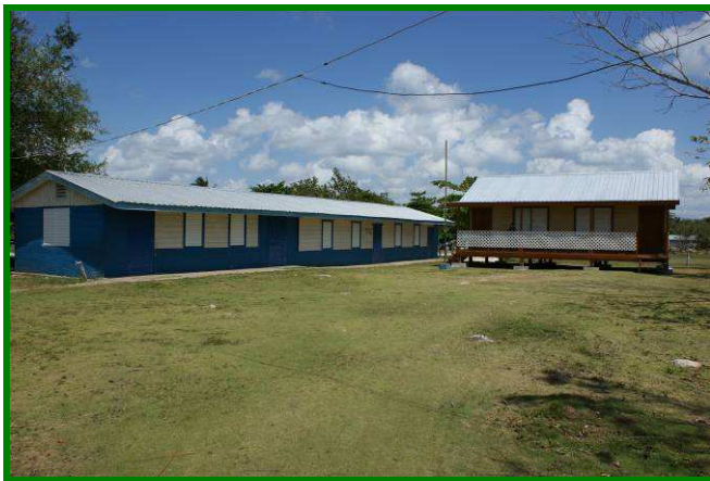
Indian Church Primary School Buildings
